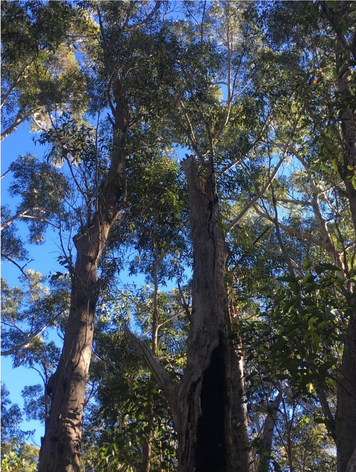
Plate J7: HBT 13 – unlikely, hollow 3m high, spout extending to secondary opening at bottom of tree
