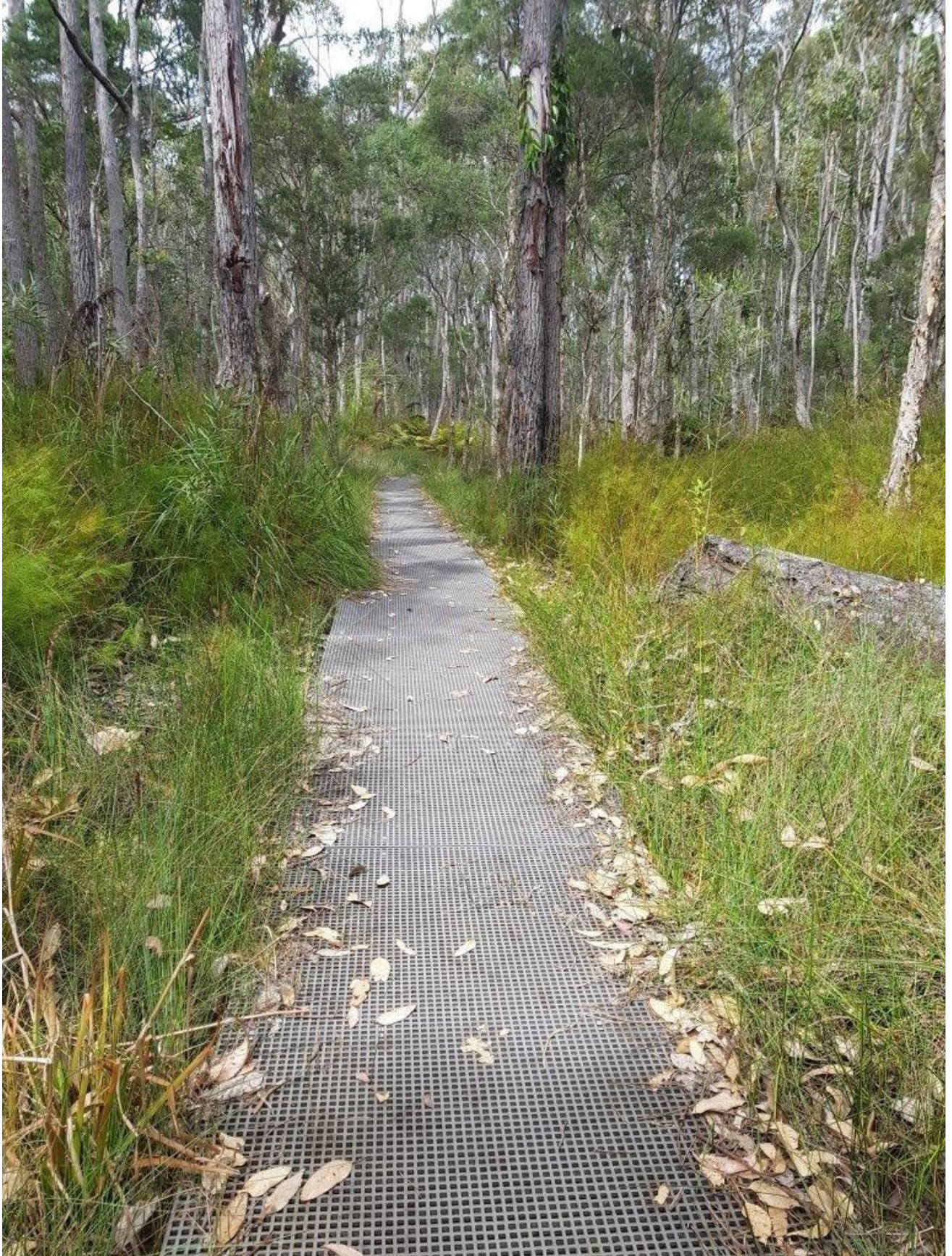
Figure 3.3: An example of a boardwalk at Garrads Reserve, Narrawallee
