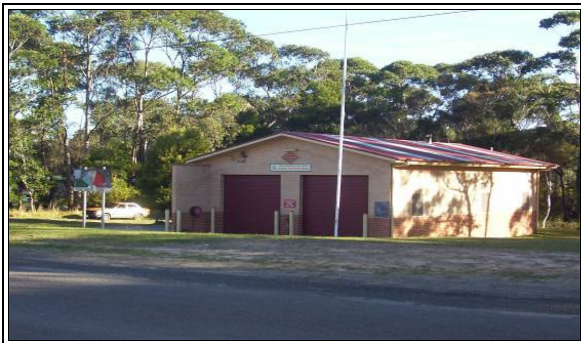
Plate 9: Existing Volunteer Fire Shed – Cunjurong Point/Manyana Brigade
