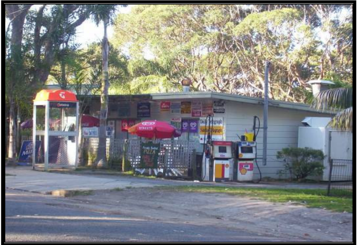
Plate 1 – Existing Shop at Cunjurong Point
