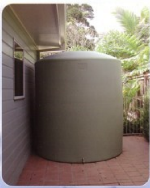
Figure 3.1: Typical Rainwater tank installation
