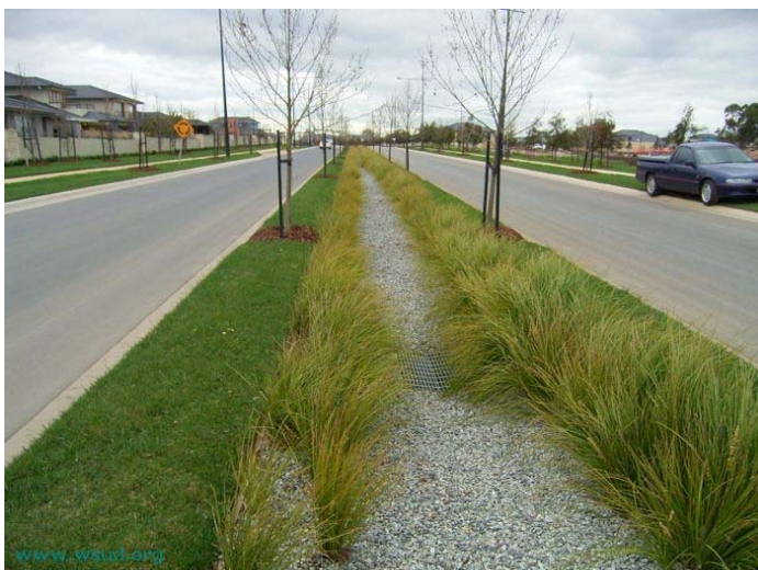
Figure 3.3: Typical biofiltration trench
